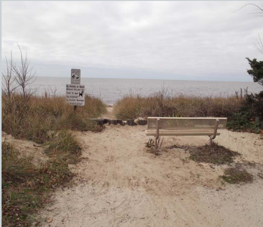
Timber Wall at Atlantic Avenue
