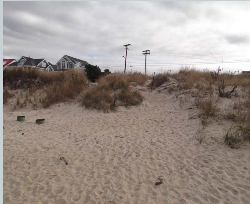
Whittier Avenue after repairs
